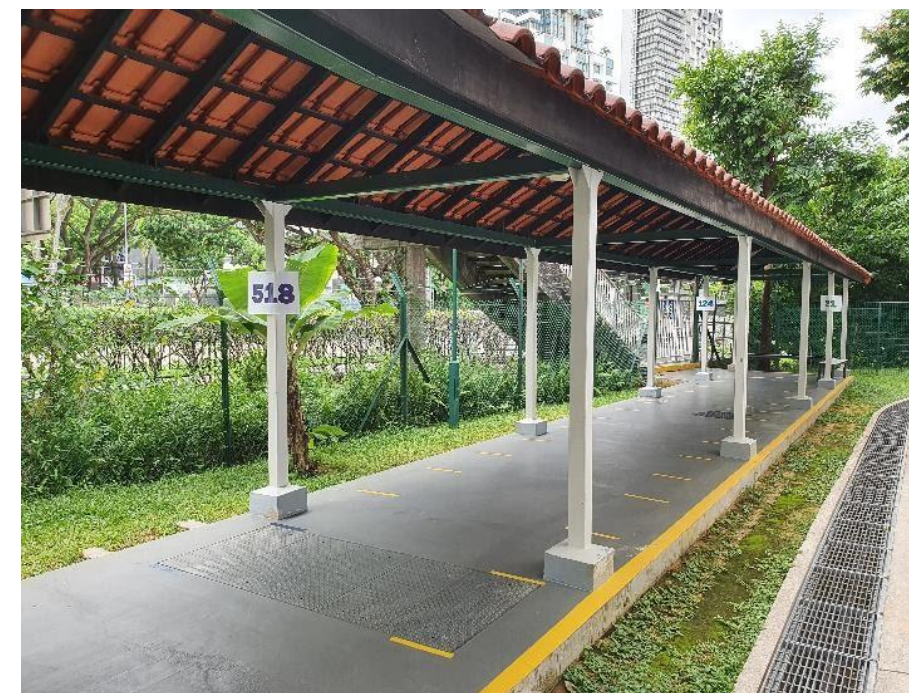
Gate 3 – Moulmein Rd
